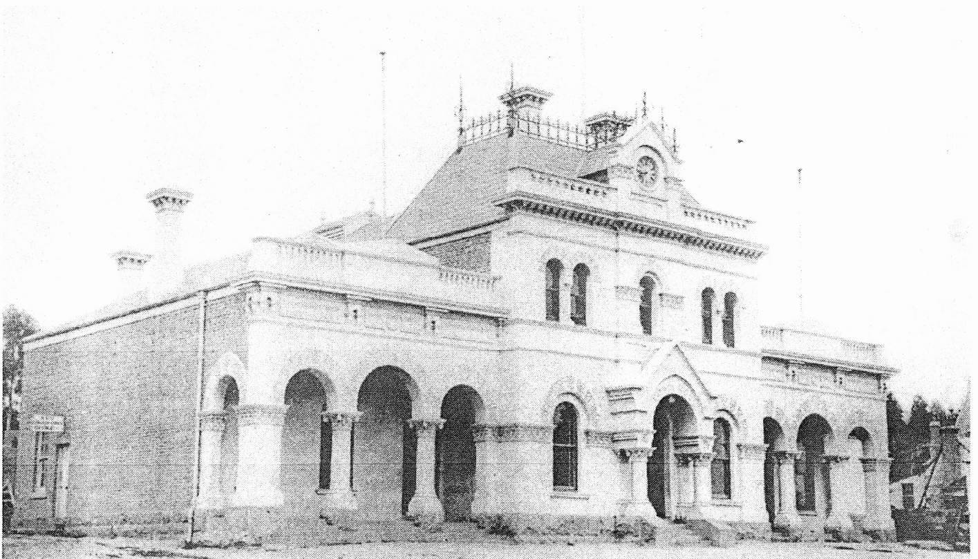
The Clunes Town Hall and Court House, an impressive monument to civic pride and progress, completed in May 1873. The chief office holder in this building, Clunes Mayor William Blanchard, played an important part in the Lothair strike and its racist aftermath.
